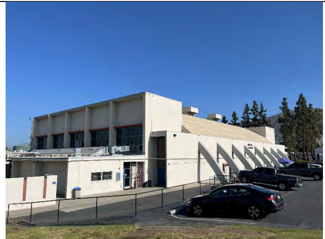
South and east elevations, facing northwest
