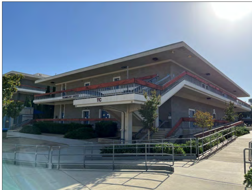
Technology Center (TC), south and west elevations, facing northeast.
