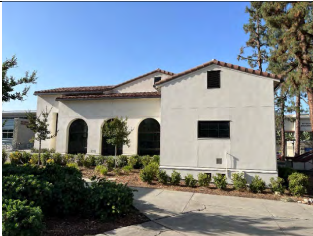
North elevation, facing south
