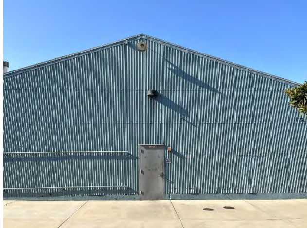
North elevation, facing south
