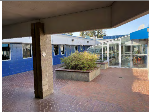
Courtyard, facing south
