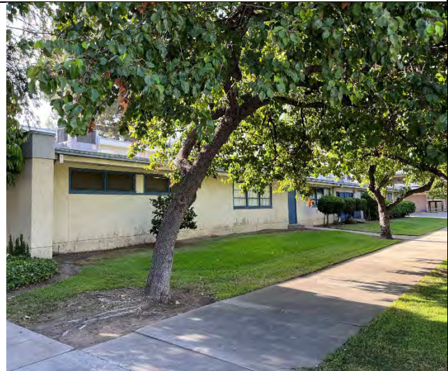
West elevations, facing southeast
