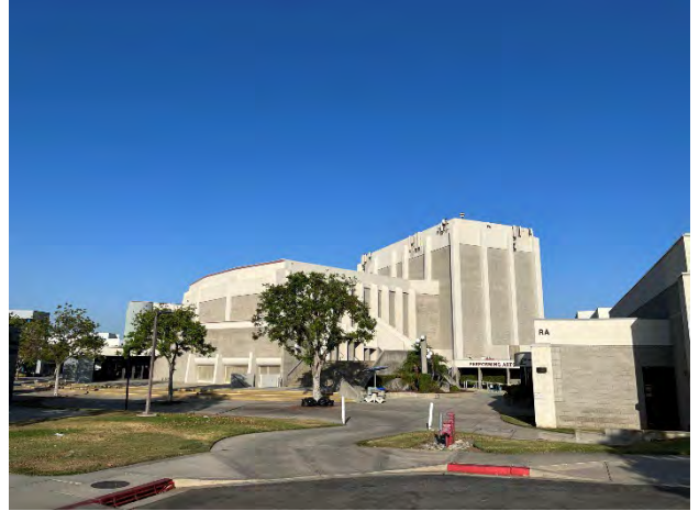
South and east elevations, facing northwest
