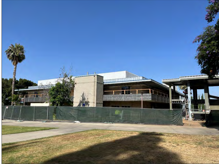
Education Development Center (ED), north and east elevations, facing southwest.
