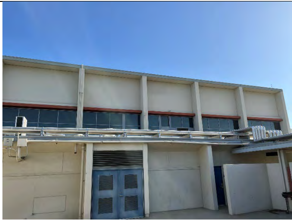
South elevation, facing north
