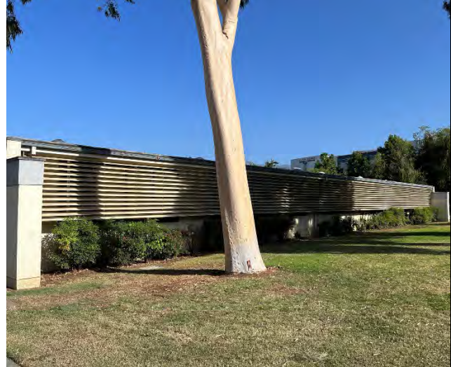
East elevation, facing northwest
