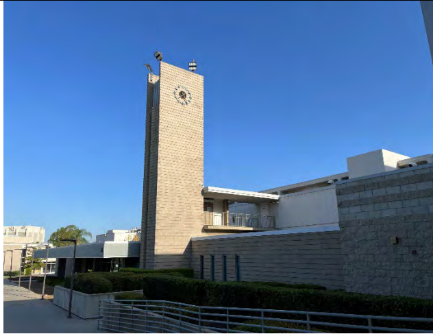
South elevation, facing northwest
