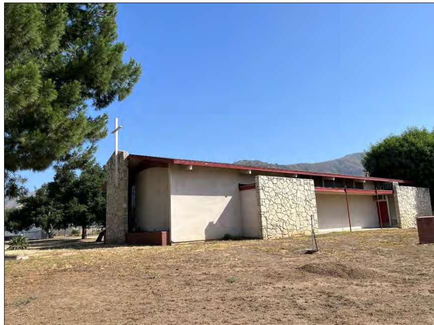
Church located at AIN 8625-022-903, south and west elevations, facing northwest.
