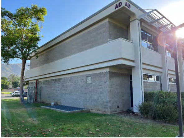
West elevation, facing northeast
