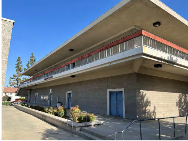
South elevation, facing northwest
