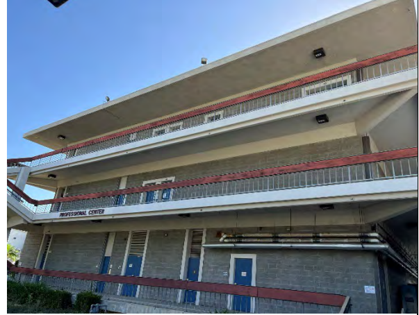
West elevation facing east
