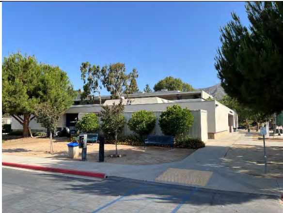
South elevation, facing north
