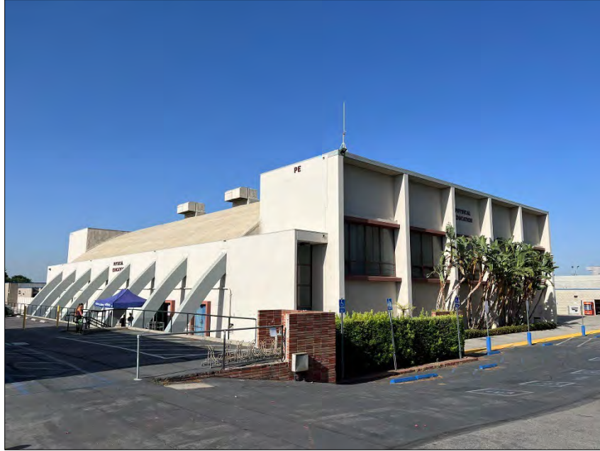
Physical Education Gym (PE), north and east elevations, facing southwest.
