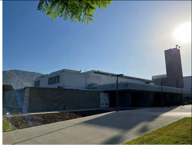
South and west elevations, facing northeast
