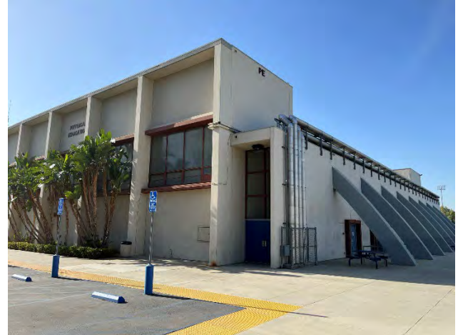
North and west elevations, facing southeast
