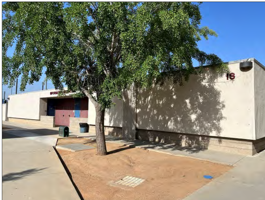
Information Services (IS), east elevation, facing southwest.
