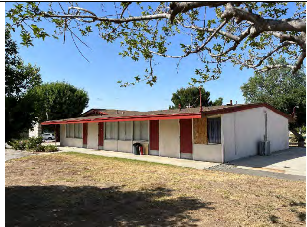
East and north elevations, facing southwest
