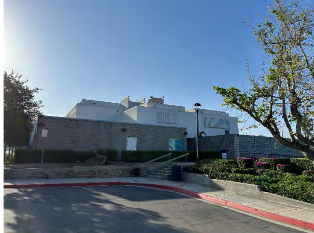
West elevation, facing east
