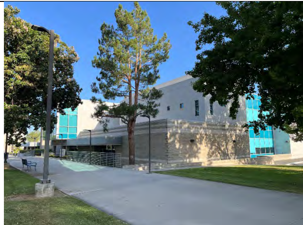
East addition, facing northwest
