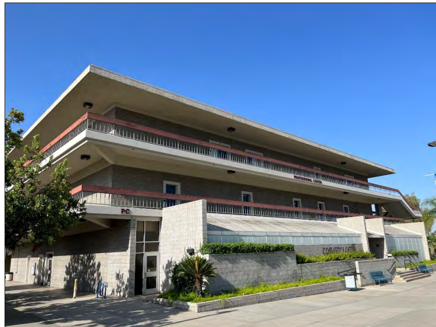
Professional Center (PC), north elevation, facing southwest.
