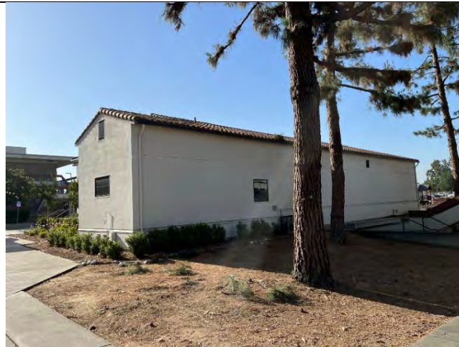
North and west elevations, facing southeast
