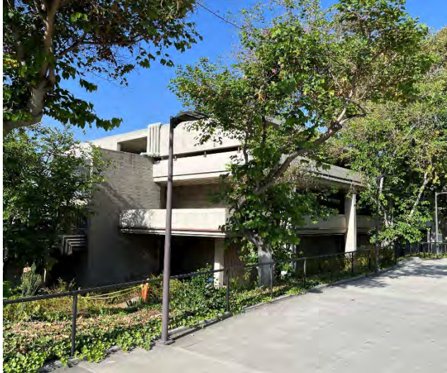
North and west elevations, facing southeast
