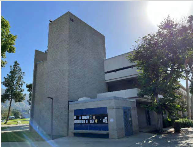
West elevation, facing northeast
