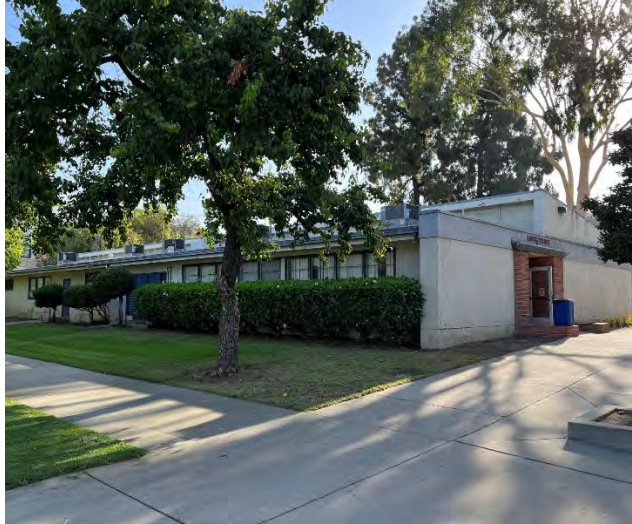
South and west elevations, facing northeast
