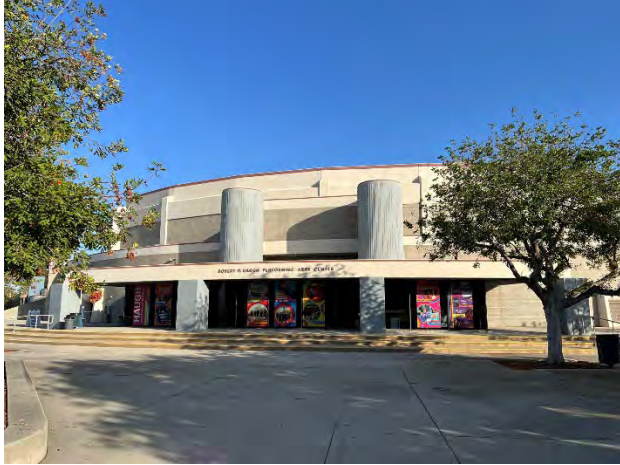
South elevation, facing north
