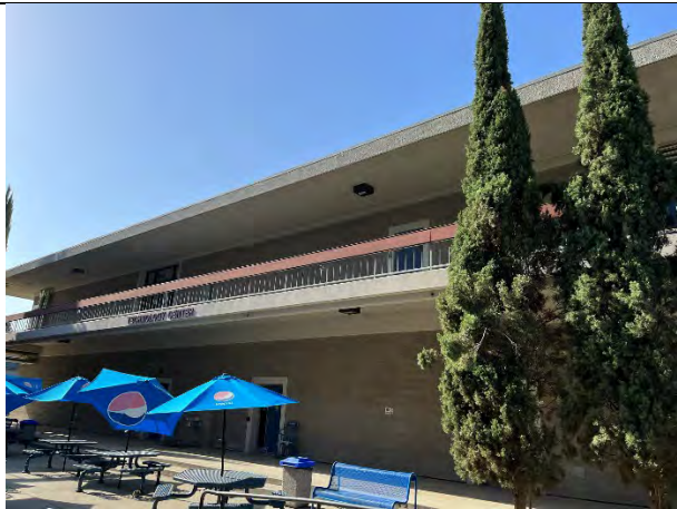
North elevation, facing southeast
