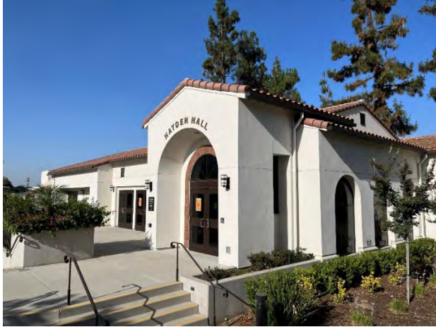
North and East Elevations, facing southwest
