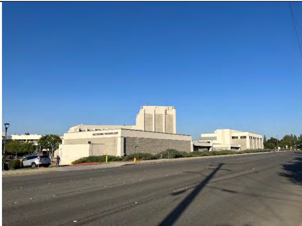
North elevation, facing southwest
