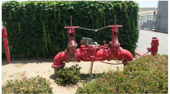
Noise Measurement Site 3 - looking south
