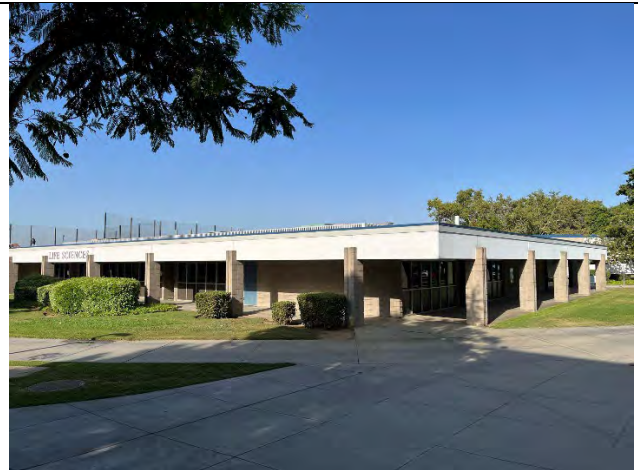
North and east elevations, facing southwest
