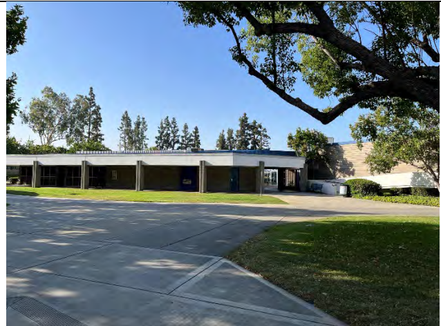
North elevation, facing south
