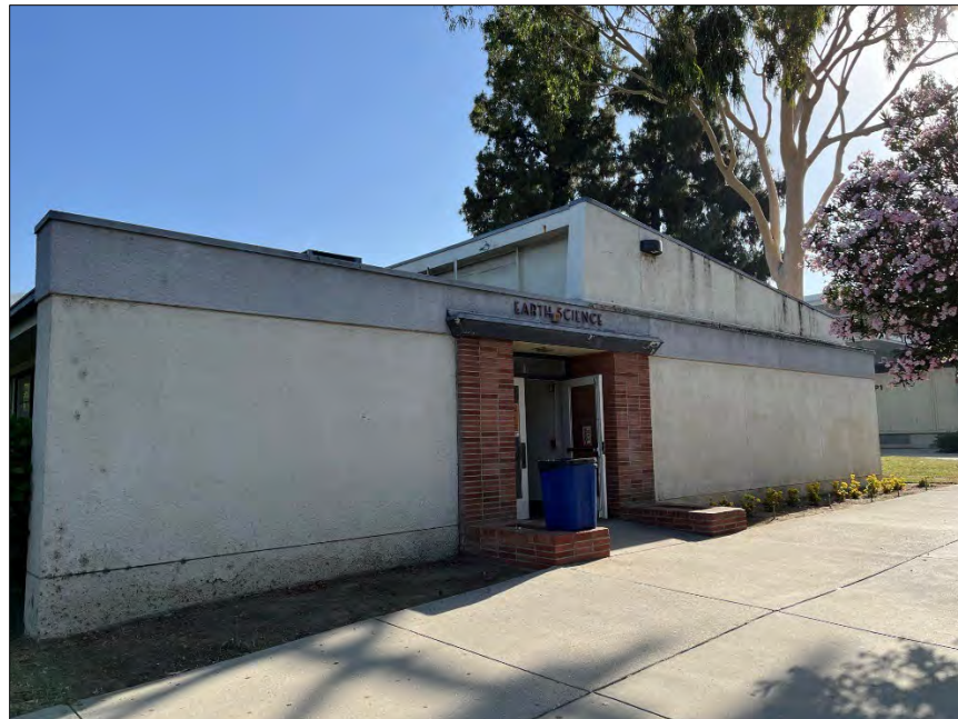
Earth Science (ES), south elevation, facing northeast.
