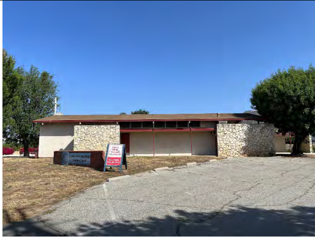
South elevation, facing north
