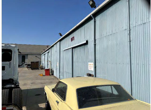
East elevation, facing southwest
