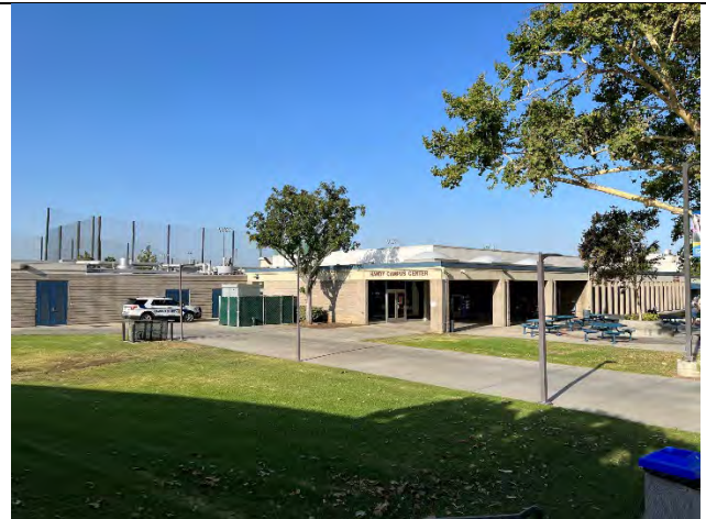
East elevation, facing southwest
