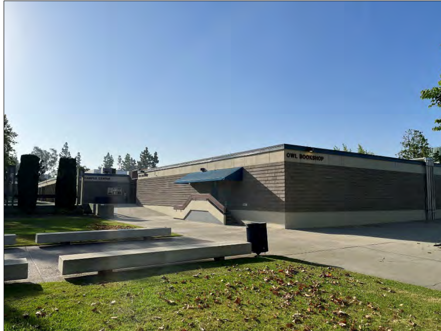
Owl Book Store/Campus Center (BK/CC), north and west elevations, facing southeast.
