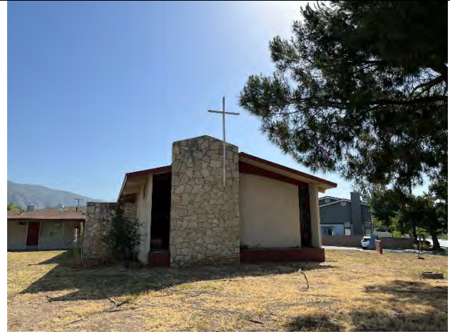
west elevation, facing east
