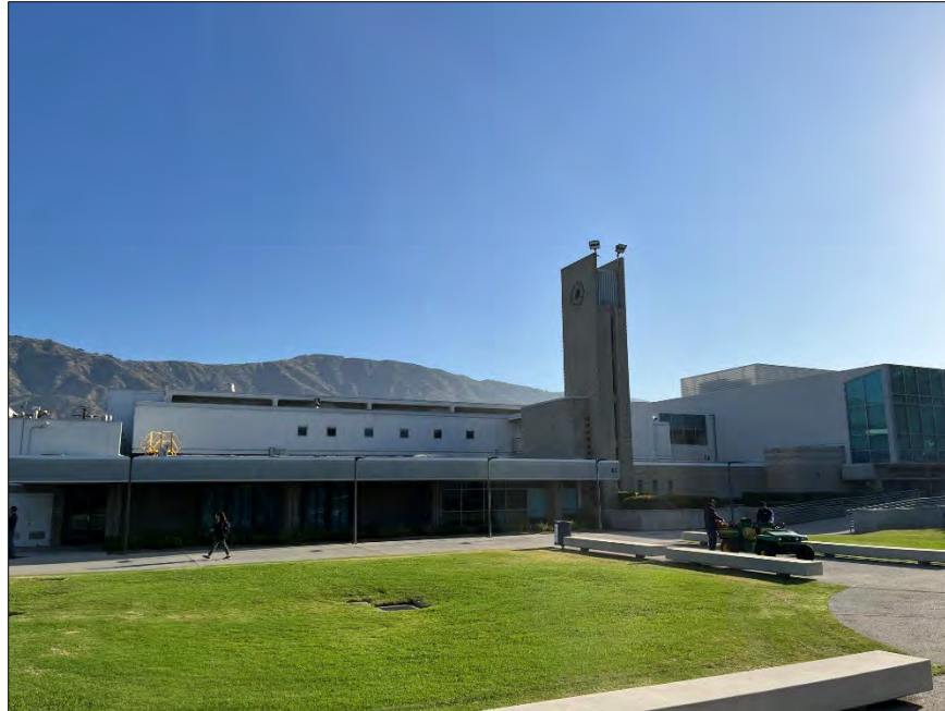
Hayden Library (LI), south elevation, facing northeast.
