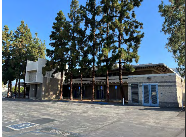
South elevation, facing north
