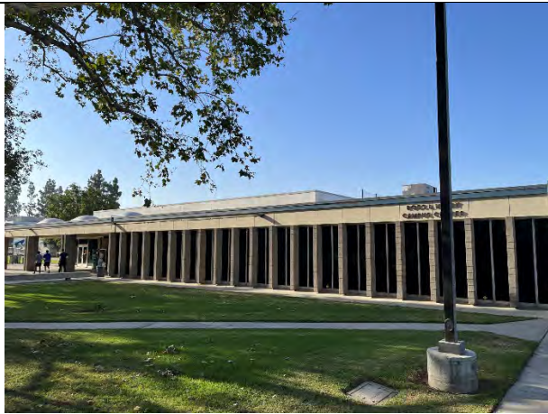
North elevation, facing southeast
