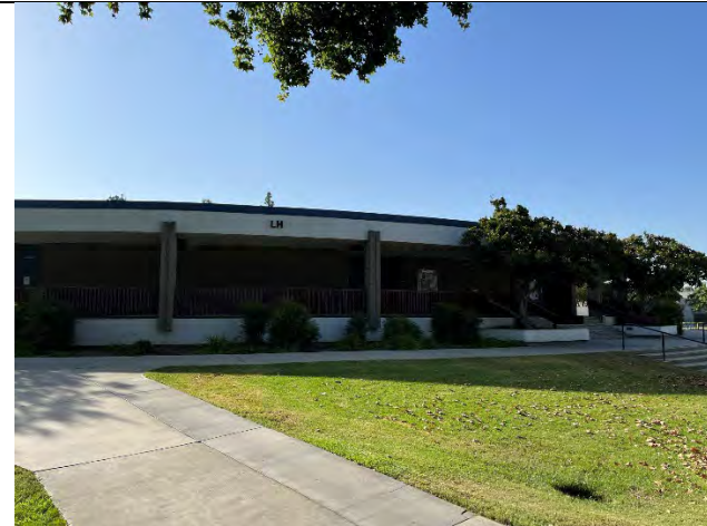
West elevation, facing southeast
