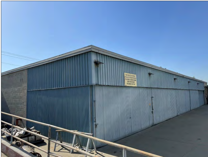
Automotive Annex (AA), west elevation, facing southeast.
