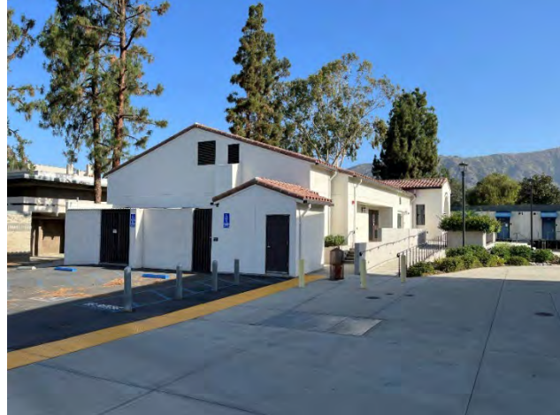
South and east elevations, facing northwest
