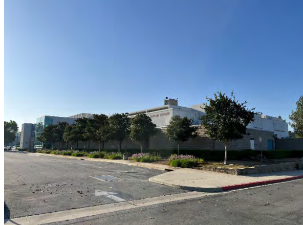
North and west elevations, facing southeast
