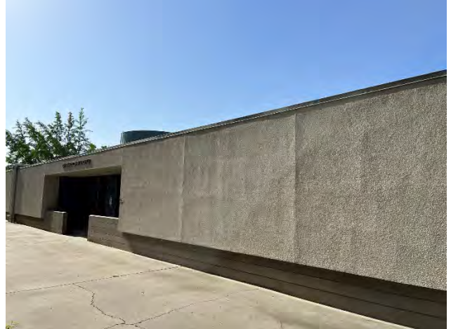
West elevation, facing northeast
