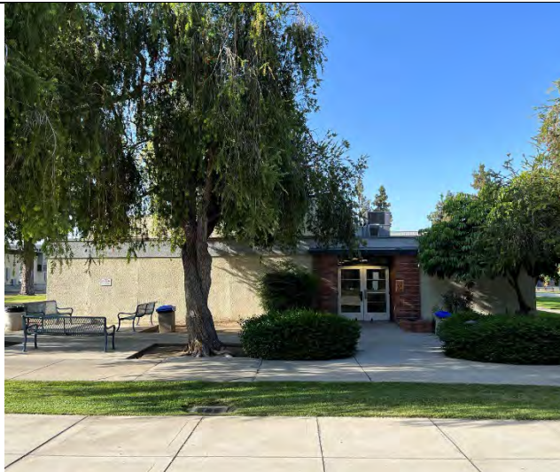
North elevation, facing south
