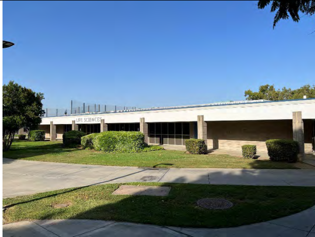
east elevation, facing southwest
