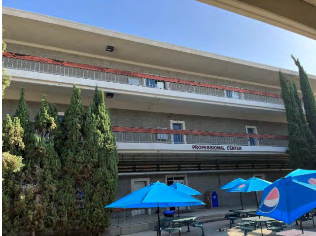
South elevation, facing north
