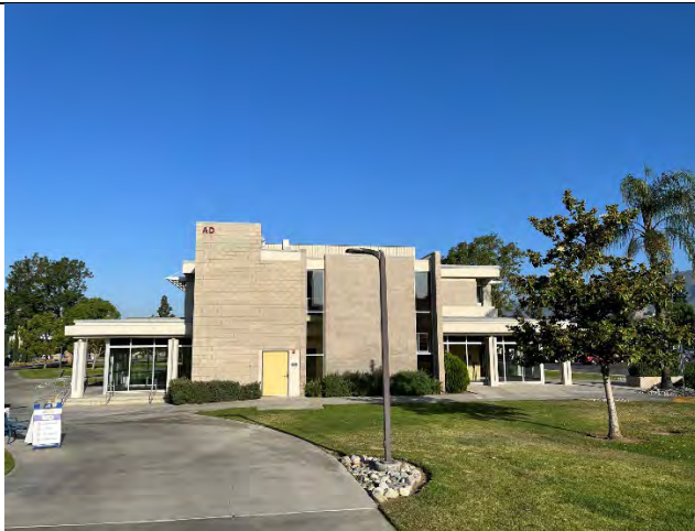
East elevation, facing west
