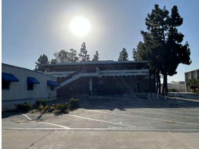
West elevation, facing east
