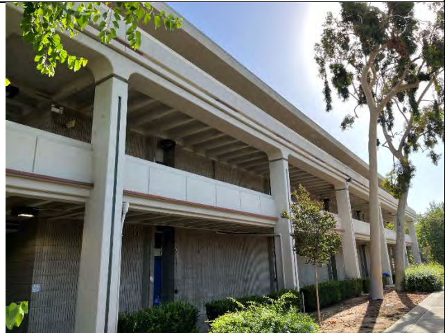
South elevation, facing northeast
