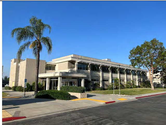
North and west elevations, facing southeast
