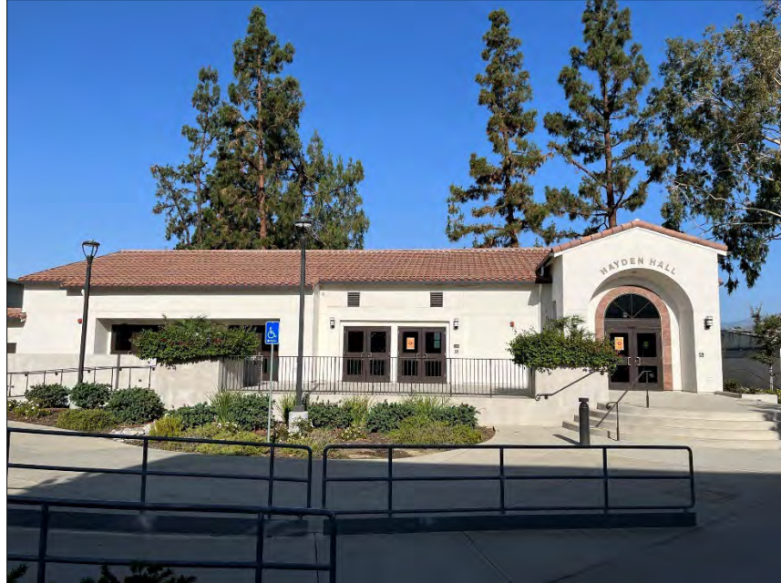
Hayden Hall (HH), east elevation, facing west.
