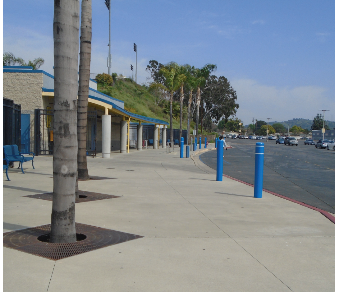
GATE HOUSE DROP-OFF / PICK-UP
