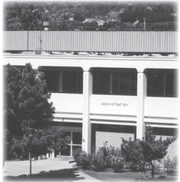
New Administration Building, opened 1967
