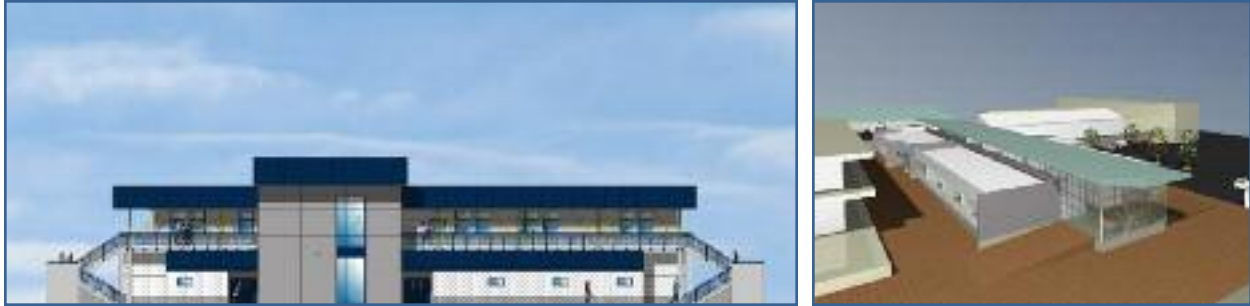
(LEFT) CONSTRUCTION ON THE FIELD HOUSE AND CONCESSION BUILDING COMMENCED IN SEPTEMBER 2007. (RIGHT) CONSTRUCTION ON THE VOCATIONAL TECHNOLOGY BUILDING BEGAN IN DECEMBER 2007.
